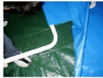
SET THE U-PIPE FRAMES INTO THE LOOPS ON THE BOTTOM OF FABRIC
